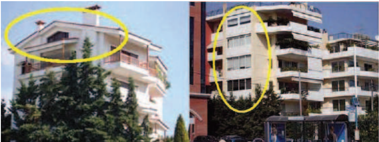
FIGURE 17: Illegal room under the roof of the building (left); Enclosure of semi-open areas that are within the ratified outline of the volume of the building (right) 46
