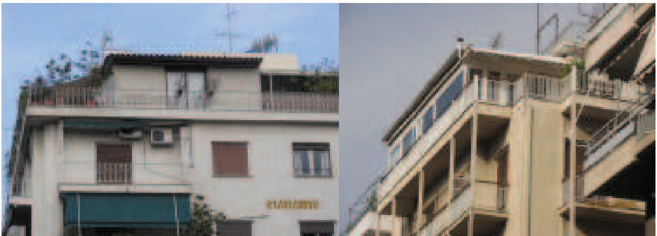
FIGURE 18: Informalities in planned areas that do not exist within the ratified outline of the volume of the building (informal closing of uncovered balconies that are not considered to be within the ratified volume), but can be formalized by Law 4014/2011
