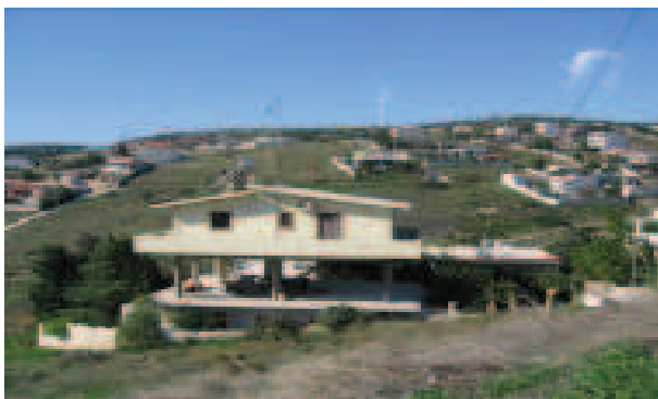
FIGURE 13: Informal buildings in unplanned areas without a permit (photo by C. Potsiou)
