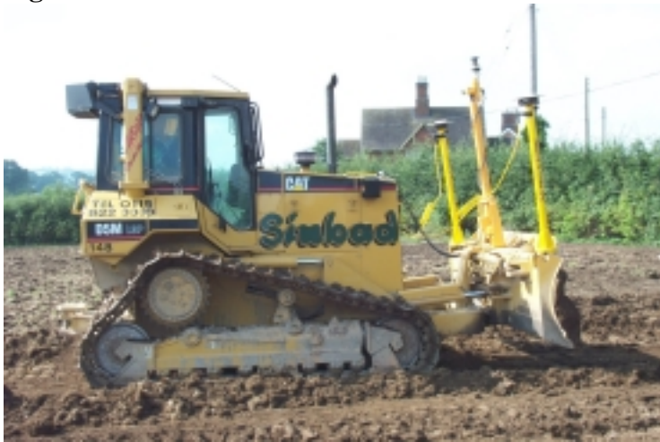
Figure 3: Bulldozer with SiteVision GPS installed
