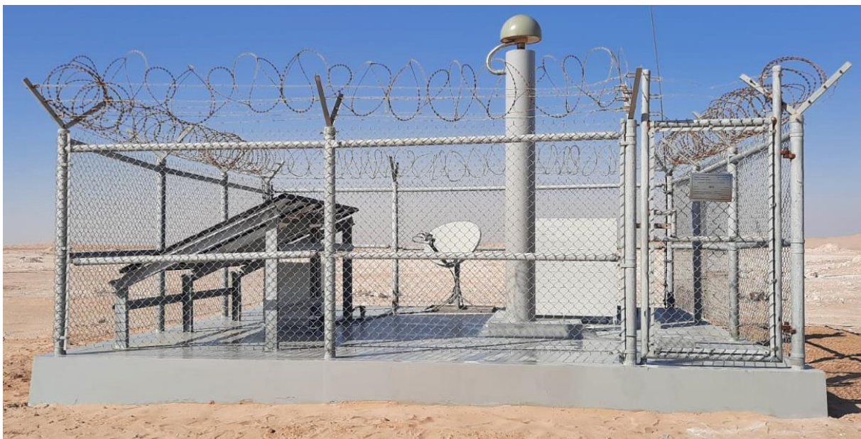
Figure 1: A typical KSA-CORS Ground Type station
