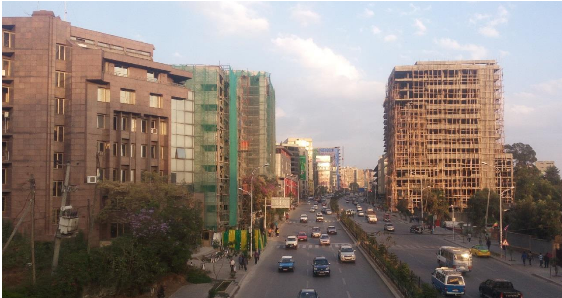
Photo 1. Construction in Addis Ababa Bole Road 2017 (photo by TH)
