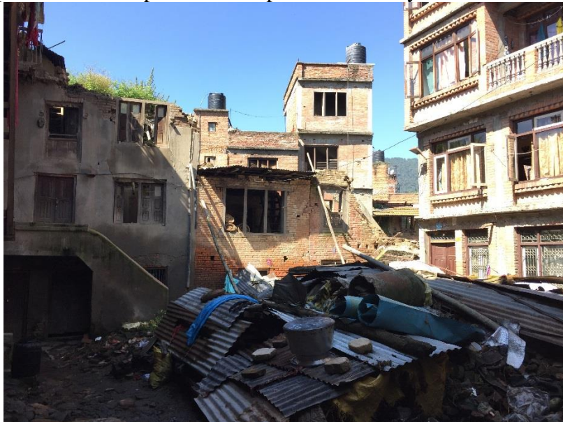
Picture 1: Damaged houses in Khokana
