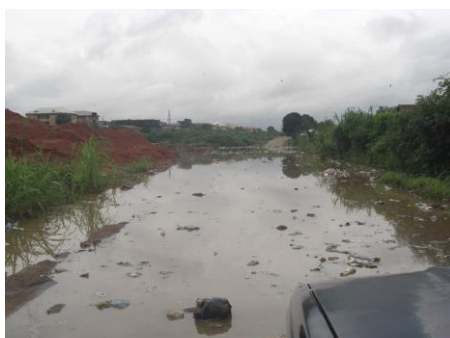
Fig. 10e Natural Flow route at Chukwuma Nwoha Road Area photographed on 20 th July 2012. The natural flow route here runs across the road from right to left. It has been blocked by the road to which this road joins.
