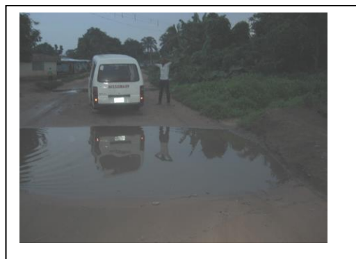
Fig. 10c Natural Flow route at Avu Owerri West L.G.A. photographed in June 2012. Buildings on the left are already blocking the natural flow routes.
