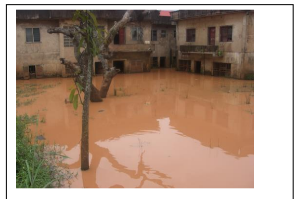
Fig. 10d Natural flow route at Works Layout Area Owerri, blocked with buildings, photographed on 6 th October 2011
