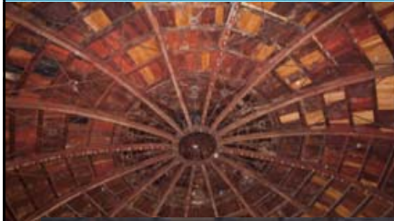
Interior view of the dome with the sixteen steel ribbings
