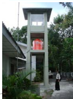
Fig. 4. (a) Design and (b) the first tower for RTS and GNSS CORS at SRM1 station, (c) Setting up of Robotic Total Station
