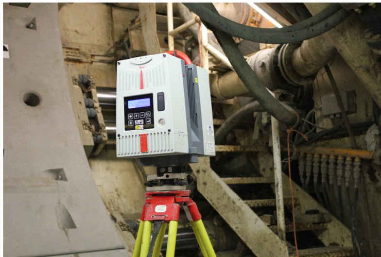
Figure 1: Scanning position in the head of the TBM
