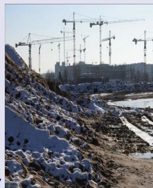
Construction of Miasteczko Wilanow in Warsaw
