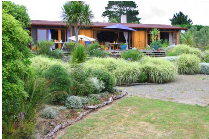
This was my own house, one of the four I had personally designed and built on the park. The solar heating unit glints in the sun but that is about it.
