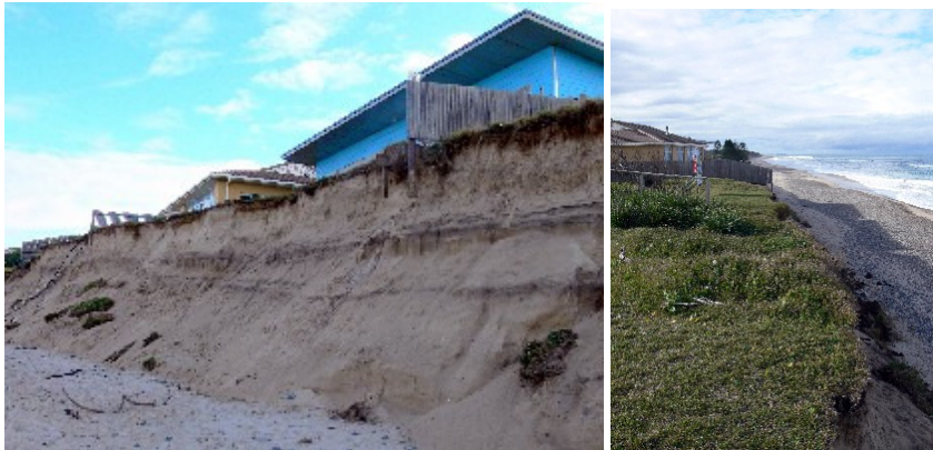
Erosion at Old Bar (New South Wales)
