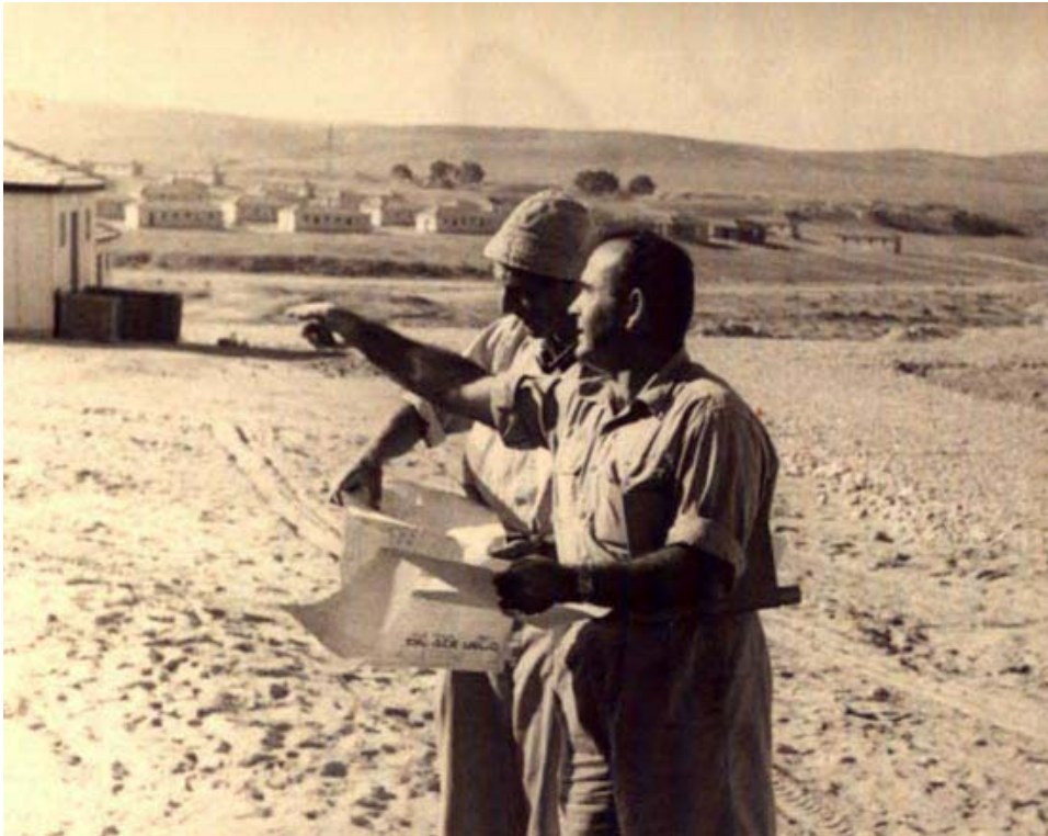
Fig. 9: Surveyors at a new building site in Beer-Sheva during the 1950's.
