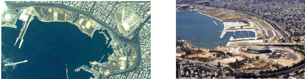
Figure 11. Infrastructure projects in Faliron area
