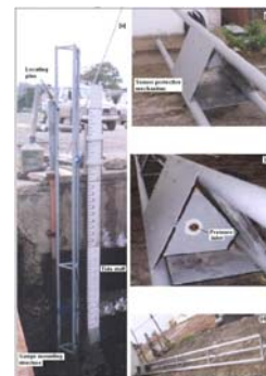
Illustration Of Sea Level Gauge Installation Details At Takoradi GLOSS Station
