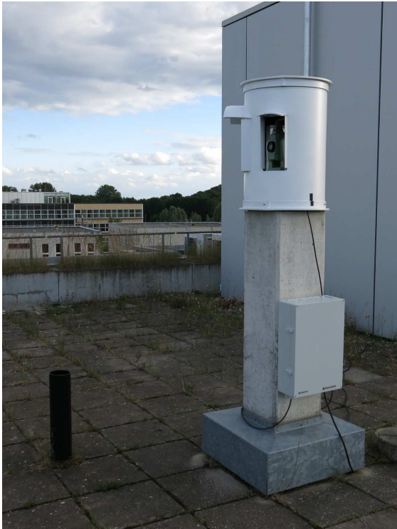
Fig. 4 Monitoring station with Leica TM30 totalstation and embedded sensor control unit, based on a Raspberry Pi
