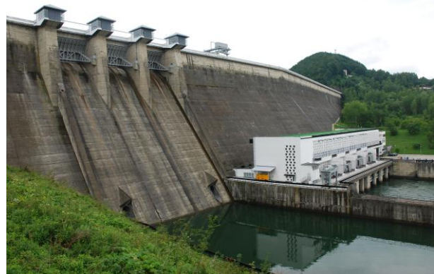
Figure 10. Heavy concrete dam in Solina
