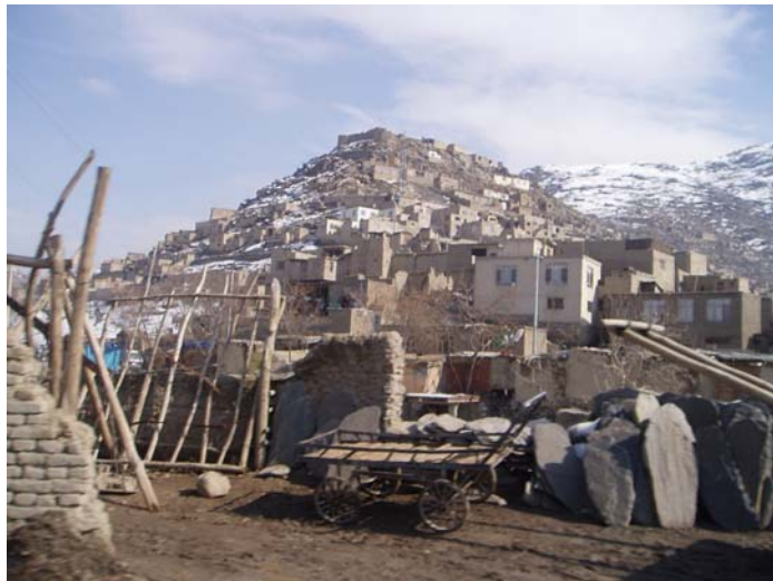
Figure 3: Infrastructure Conditions in Parts of Kabul
