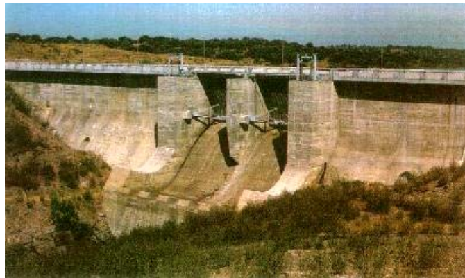
Figure 1: Monte Novo dam
