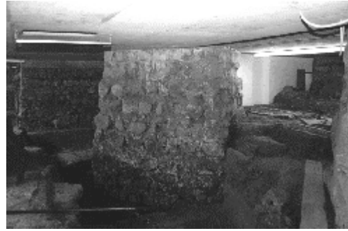
Figure 7 Cologne Cathedral underground view
